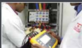
LOAD FLOW & HARMONICS ANALYSIS
